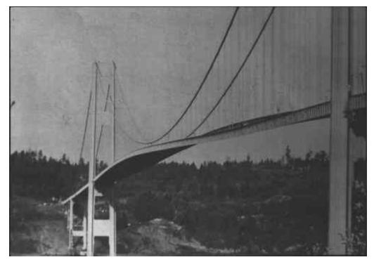
The picture above is the Tacoma Narrows Bridge shortly before it collapsed. A moderate wind initially excited small ripples that grew into violent oscillations. Eventually, these tore the bridge apart. This was a spectacular case of resonance.
